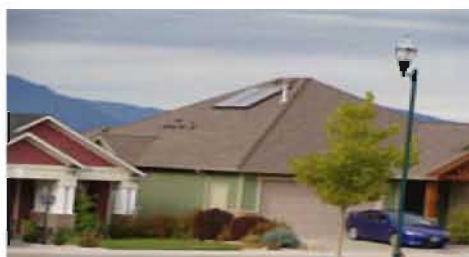
Roof Mounted residential unit.
